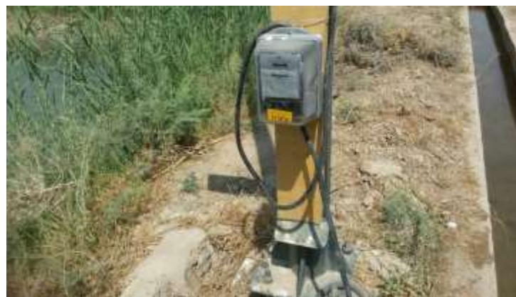
Figure 2. The counter used for measurement of energy consumption
